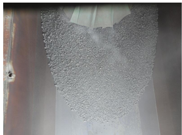
This photograph shows one Chute loading the Clinker into the hatch of a truck. The dust-control of the system is of particular note in this photograph. Cement Clinker is a very dusty, problematic product, and with the use of the Cascading technology, the emissions are greatly minimised during loading.
