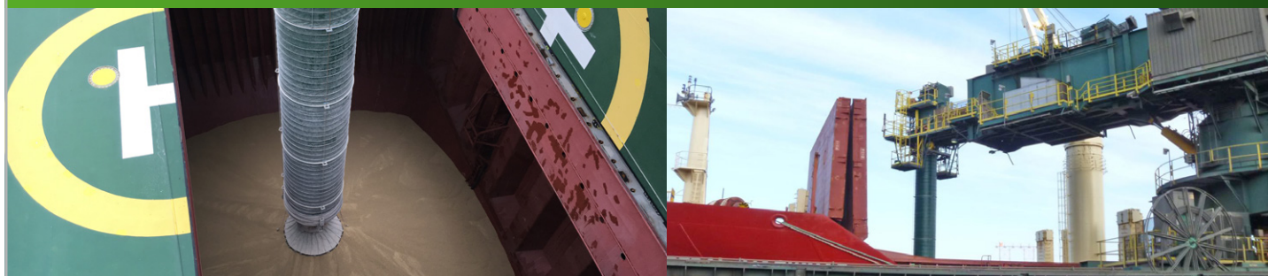
Above left: Cleveland Cascades Shiploader Loading Grains - USA Above right: Cleveland Cascades Cascade Shiploader – Metal Concentrates, Sorel Tracey, Canada.
