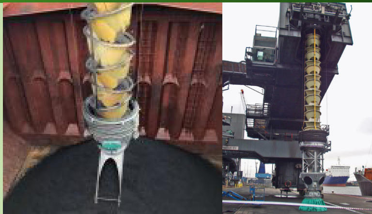
Above Left: Cleveland Cascades Shiploader Loading Coal - Columbia Above right : Cleveland Cascades Cascade Shiploader – Petroleum Coke, Immingham, UK.
