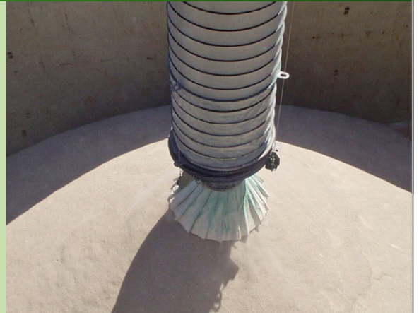
Above: Cleveland Cascades Cascade Shiploader – Bentonite.
